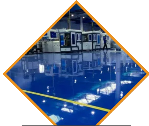
Epoxy Flooring Solution Dhaka, Bangladesh
